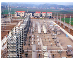
3 Gorges Dam, site of Longquan, China.
